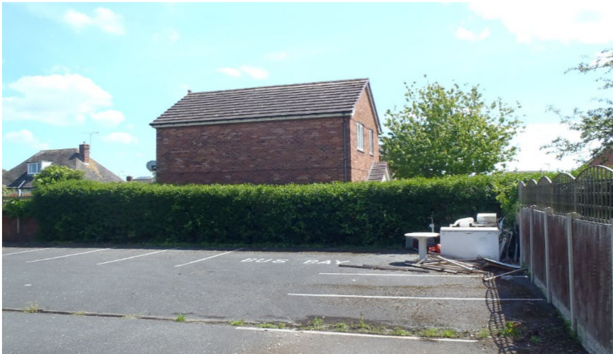
7. Looking from site to Rear – Dwelling off Cae Gruffydd LHS back
