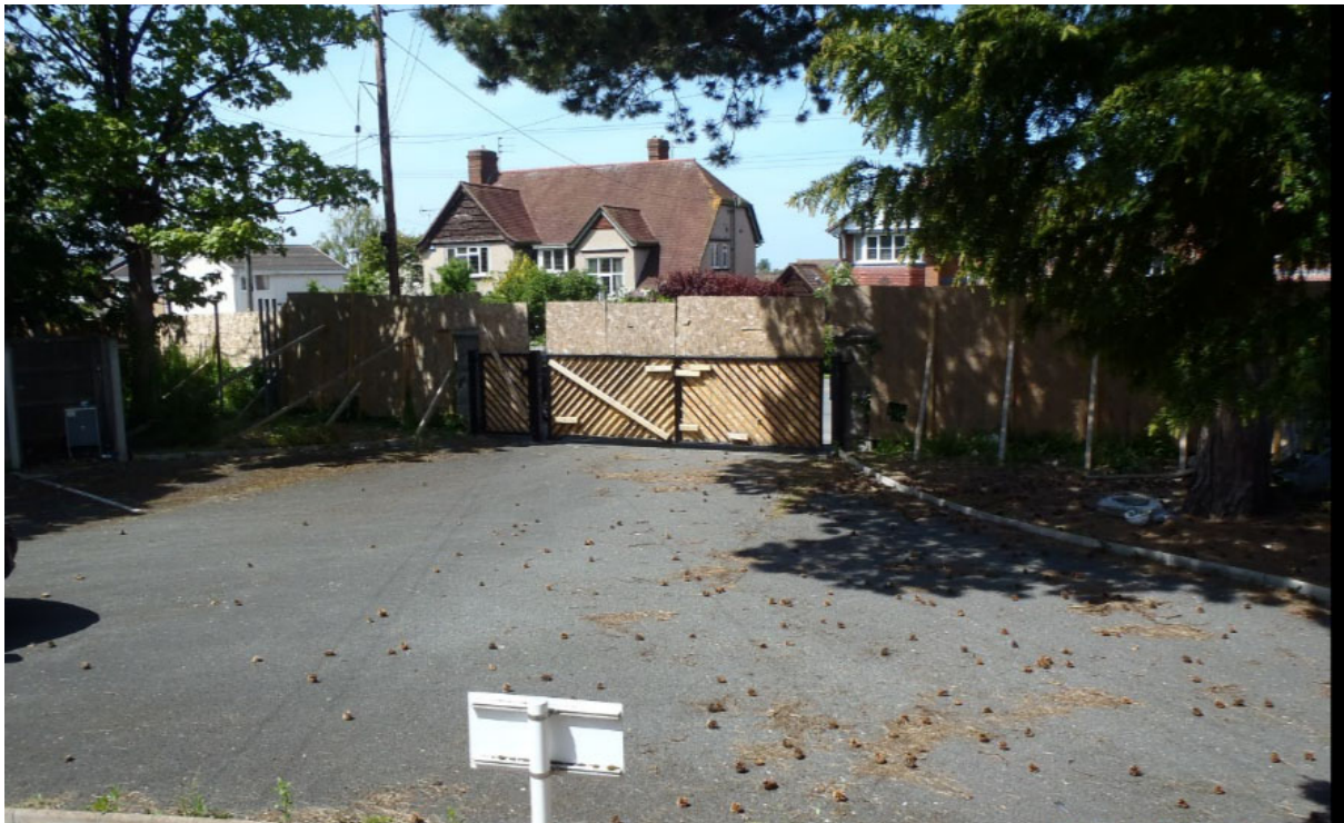
10. View from within site looking out to road; gate and temporary hoardings
