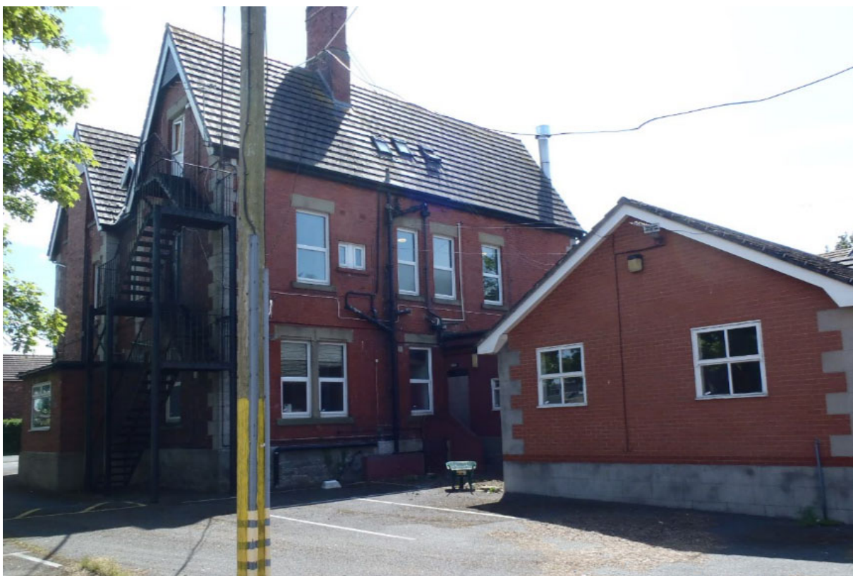
8. Side elevation; stairwell proposed to be enclosed
